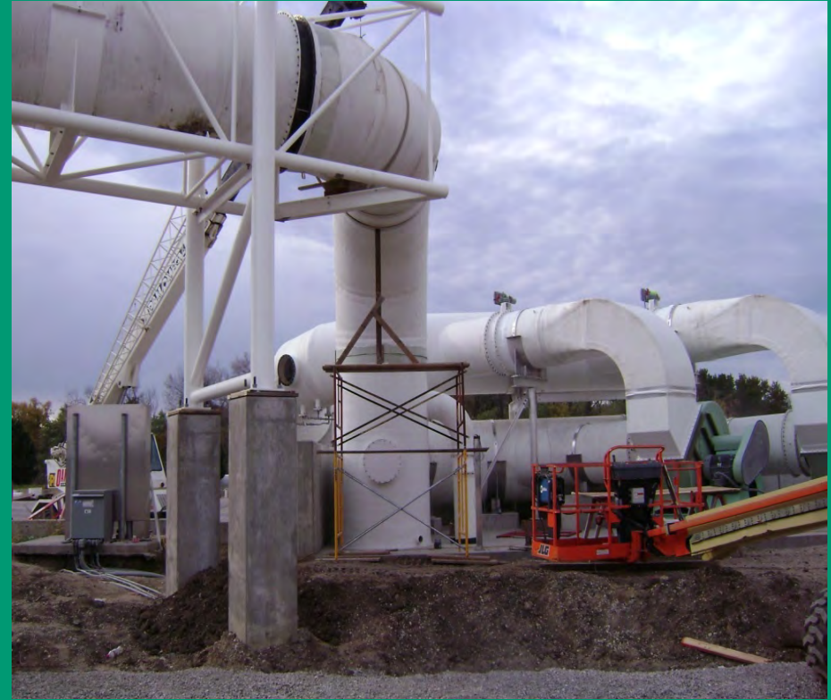
Odor Control FRP Duct – Des Moines Wastewater Treatment Plant
