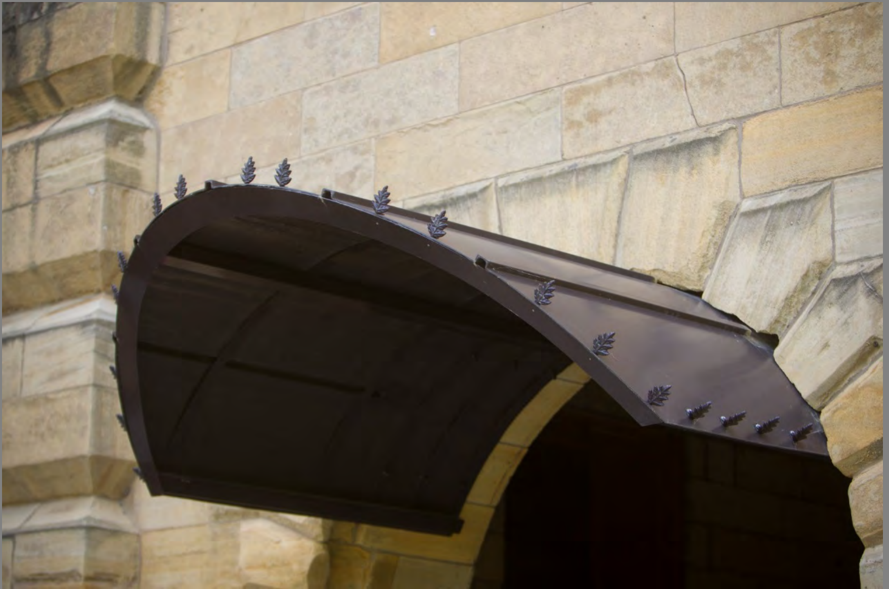
Rock Island Arsenal FRP Canopies
