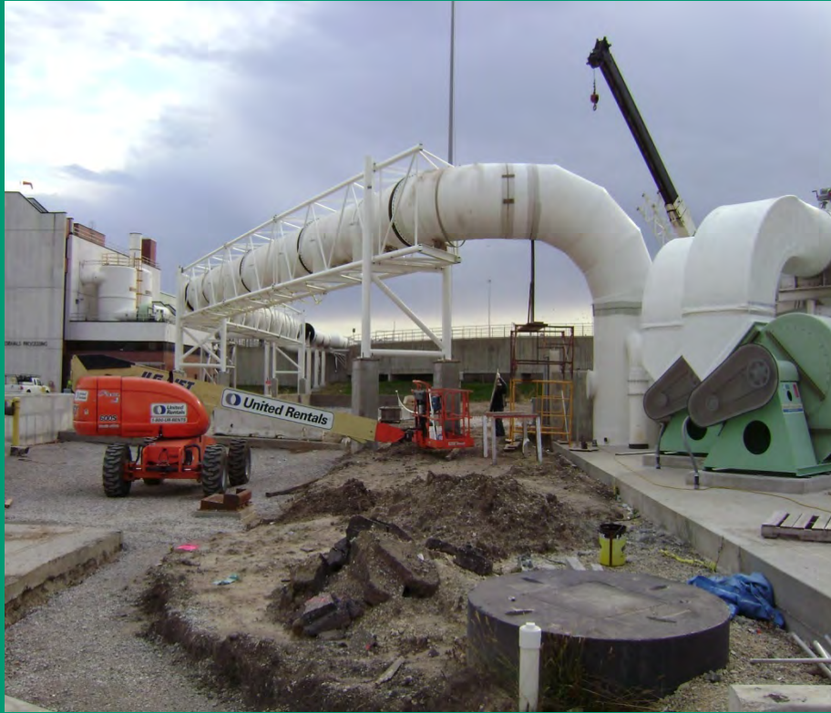
Odor Control FRP Duct – Des Moines Wastewater Treatment Plant
