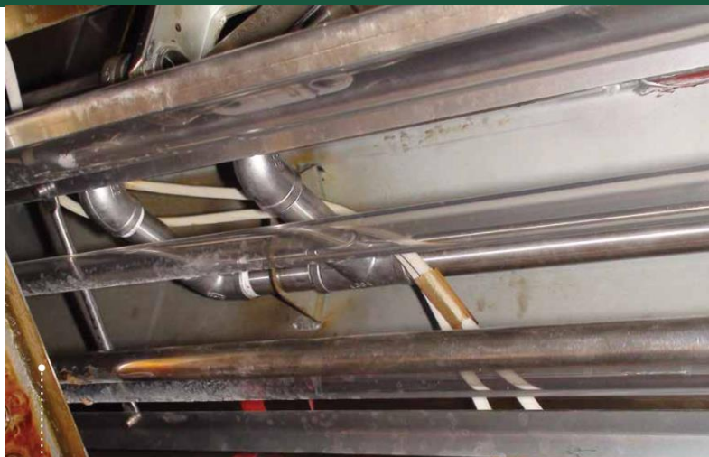
Hood with JIMCO UV-C Technology - not cleaned for 6 months
