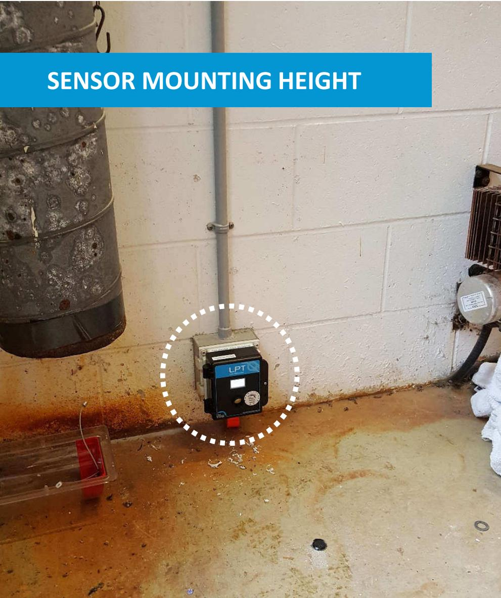
Heavier than air gas sensors should be placed 6 – 12 in / 15 – 30 cm from the floor
